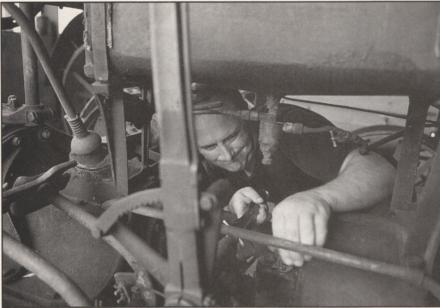
Getting down to the restoration work.
